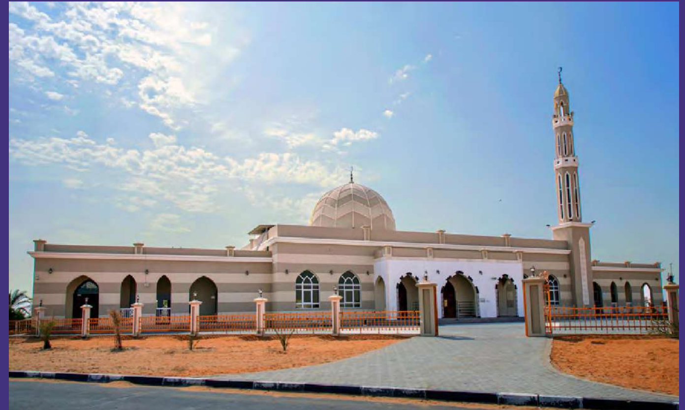
MOSQUE, Baniyas, North Abu Dhabi, UAE
