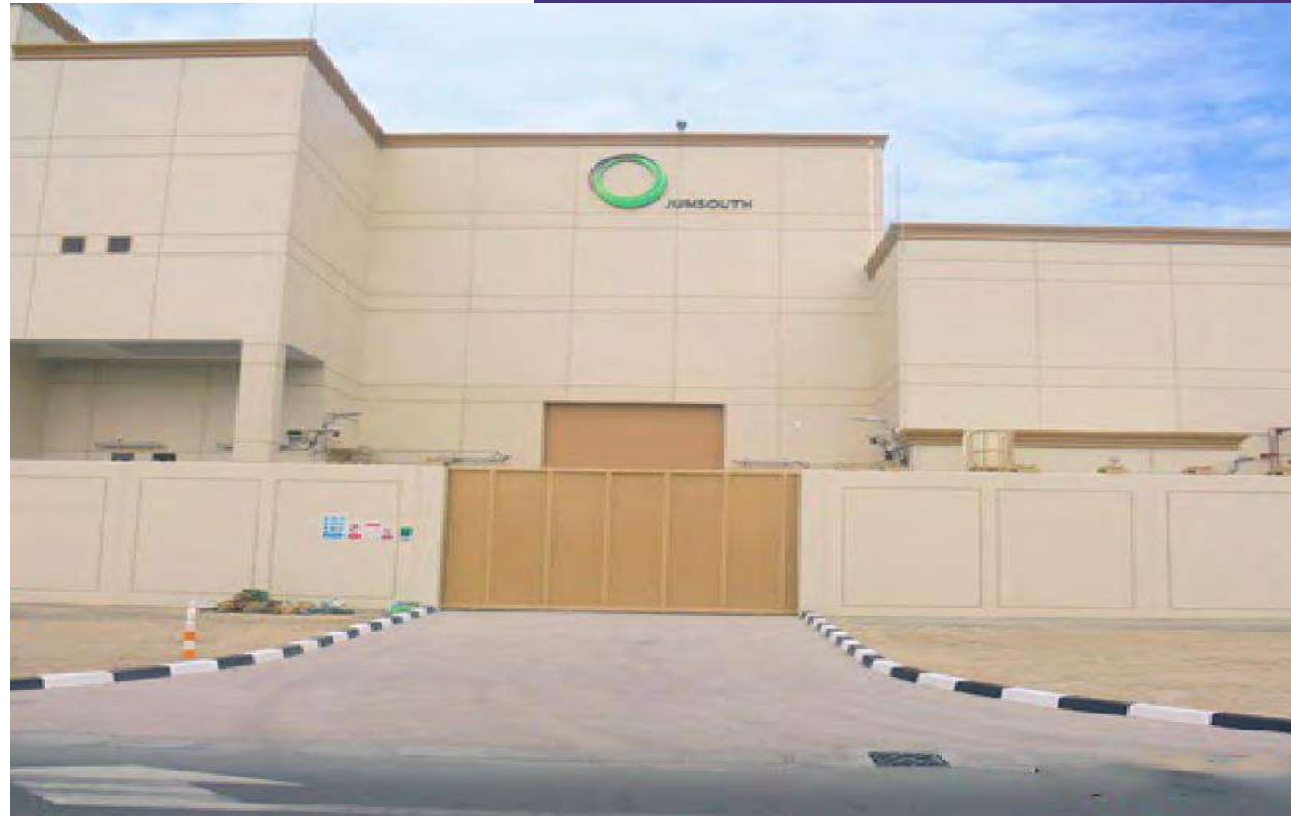
Tlal Tanya 132/11 KV Substation, Tlal Tanya, JebelAli, Dubai
