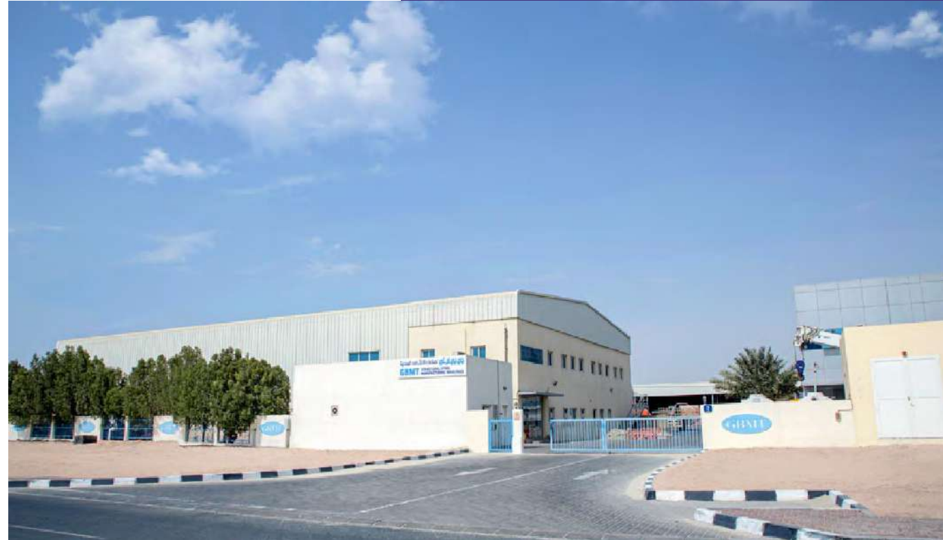
GBMT Steel Factory, ICAD III, Abu Dhabi, UAE
