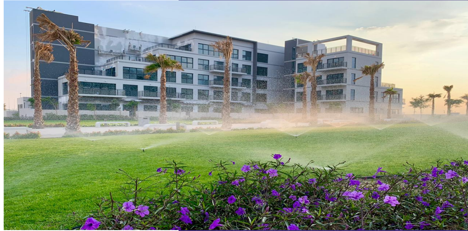
B+G+4 Residential Building, Dubai Studio City, Dubai, UAE - A, B, C, D, E
